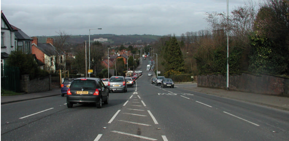
A55 Knock Road eastbound (existing)
